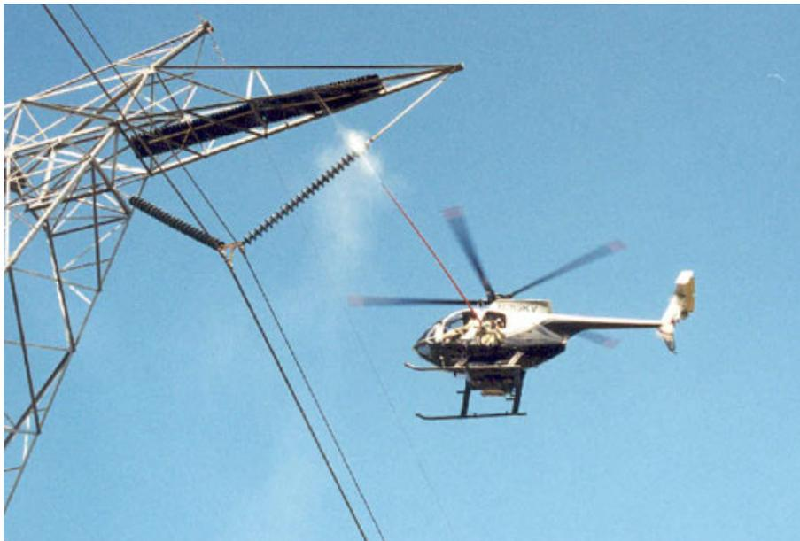
Figure –11: Washing of V- string using Helicopter.
