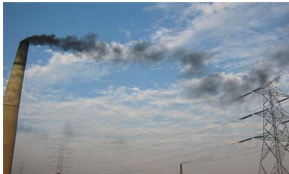
Fig-3a: Smoke from Brick Kilns polluting Transmission Line
