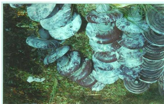
Fig-5: Deposits On Insulator Surface Due To Bird Droppings
